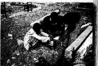
Fixing coupling at pillar top end
