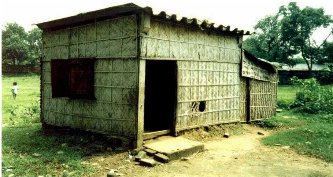
Photograph 4: Housing & Building Research Institute's model house in Dhaka. The house has a precast concrete frame and precast ferro-concrete roof but costs 15,000Tk, nearly 8 times the price of a similarly sized thatched bamboo house.
