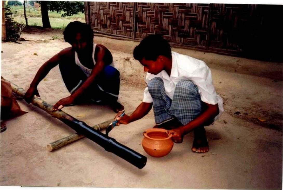
Photograph 7: Painting bitumen on bamboo posts is a cheap and effective way of making them last longer. Frequently old and rotten posts are a significant factor in house collapses during strong winds (Workshop 4: Building with Bamboo).
