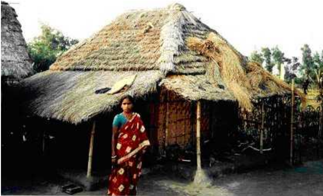
Photograph 1: A typical thatched house in Sundarban village. The main verandah (to the left of the picture) is used for eating and resting. A storage space has been created by extending the plinth to the right of the house and sheltering it with a side verandah.
