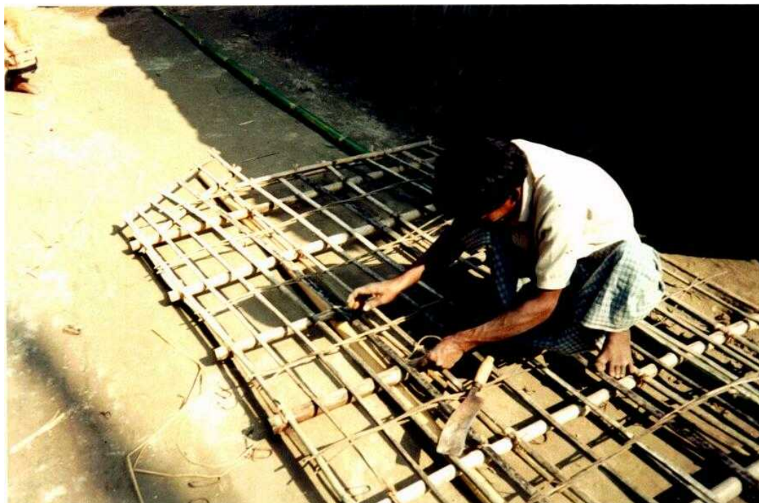
Photograph 14: Thatching frames made of bamboo and tied together with jute string all follow this particular pattern characterised by twist of green bamboo (sepni).
